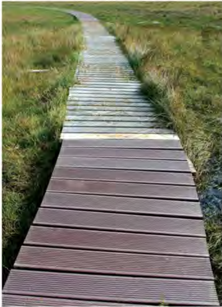
Boardwalk through peatland, Islay, Hebrides, Scotland, built of wood and recycled plastic lumber. Photo © Erik Kiviat
