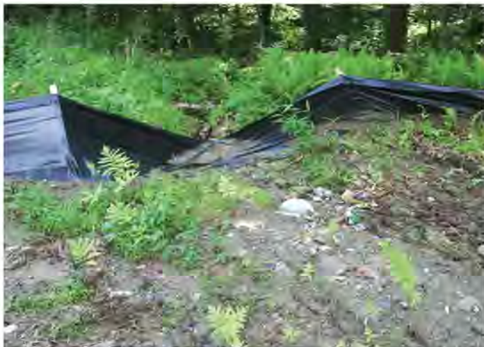
Failing or inadequate silt fences are common on construction sites, and lead to much siltation damage of streams, wetlands, and other habitats. Photo © Erik Kiviat
